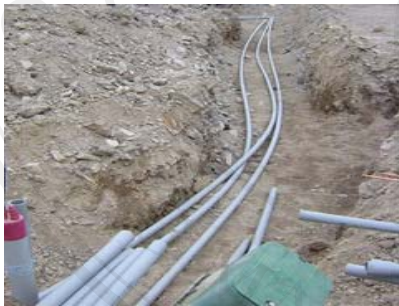
(a) cable laid in groove
