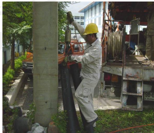
(b) pulling of cable in duct
