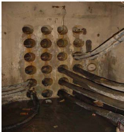
(a) internal view of manhole and duct
