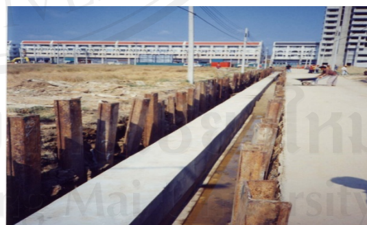
(b) concrete encased ductbank
