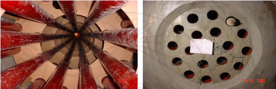
(a) arrangement of ducts in concrete pipe
