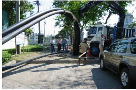
(b) pull back of polymer ducts
