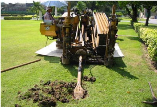
(a) drilling machine
