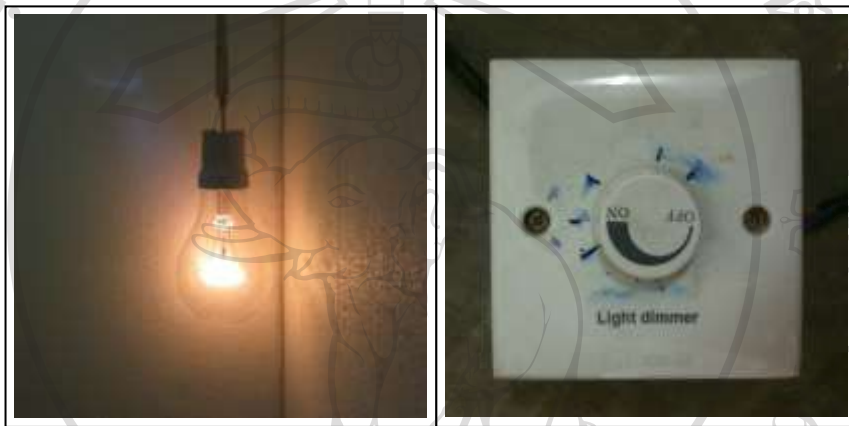
Figure 2.6 A 200-W light bulb and a dimmer-switch controller
