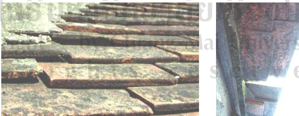
Fig.3.52 Mosses grow on the top surfaces of Liet tiles.
