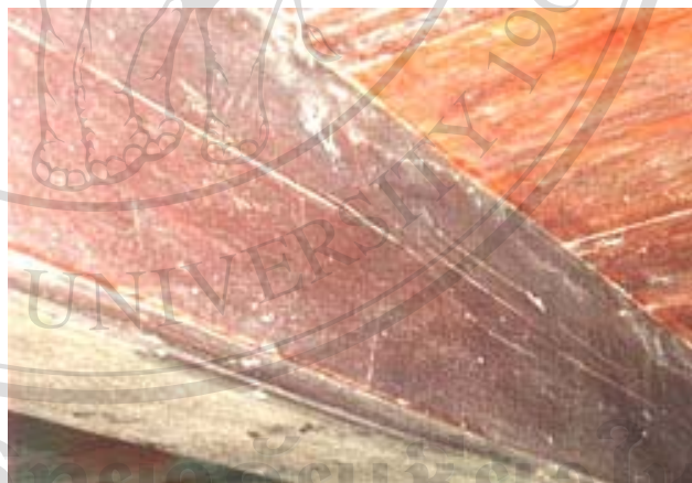
Horizontal shear against bend between grains
