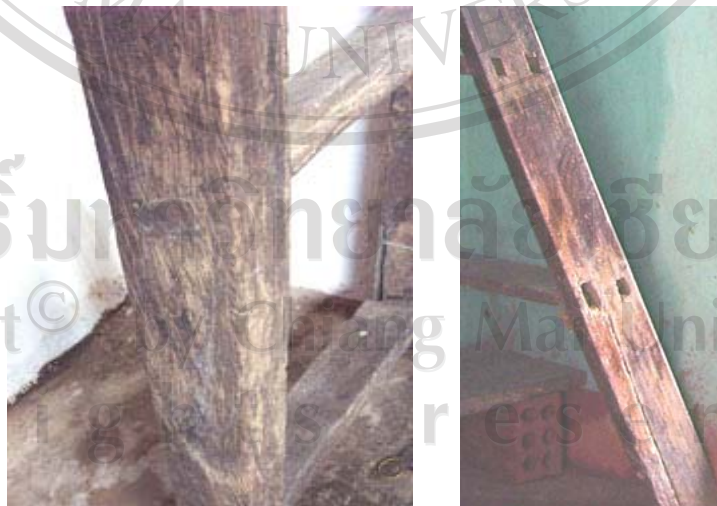
Fig.3.38 The aging process of wood and fungal attacks on their surfaces.
