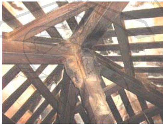
Fig.3.53 Mould and fungi on the surfaces of Liet tiles due to high moisture content inside the house.
