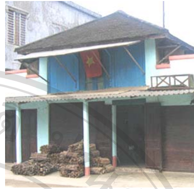
A Tu Giac house with 3 walls enclosing 3 sides except for the front side covered by wooden bars
