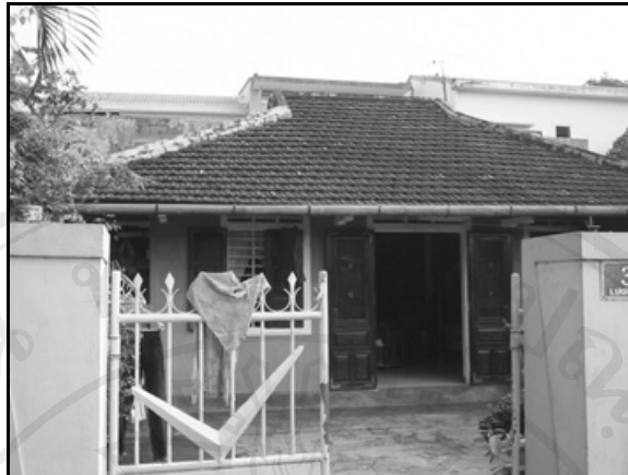
Figure 6-16: Newly built two-storied Nha Phu hid by Nha Chinh and greenery in HTGH A19
