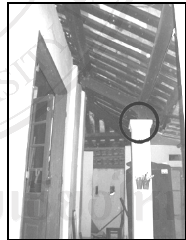
Figure 6-20: Tron Cot in veranda columns
